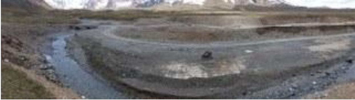
*Figure 30: Muz Tor River Borrow Area – Note regrading on far bank, levelling foreground*
