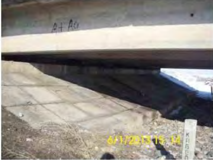
Fig. 5: An example of bridge slope protection for Kara-Unkur river bridge.
